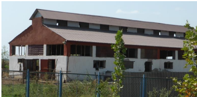
The barn with extra air inlets made by the owner.
